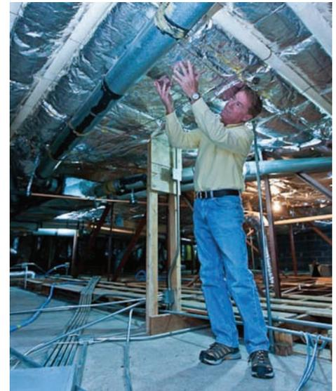
John Evans, Alpine Bank facilities officer, reviews work from a large insulation and air sealing project that improved the roof insulation factor from a leaky R-11 to a tight R-49. Photos by Todd Patrick
