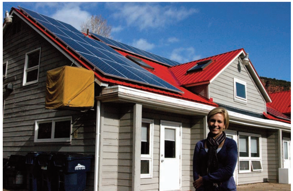
Dana Peterson stands outside Mountain Valley's main building in south Glenwood Springs. The solar-electric system on the roof is helping Mountain Valley use its greenhouse for longer, helping clients. Photo by Cam Burns
