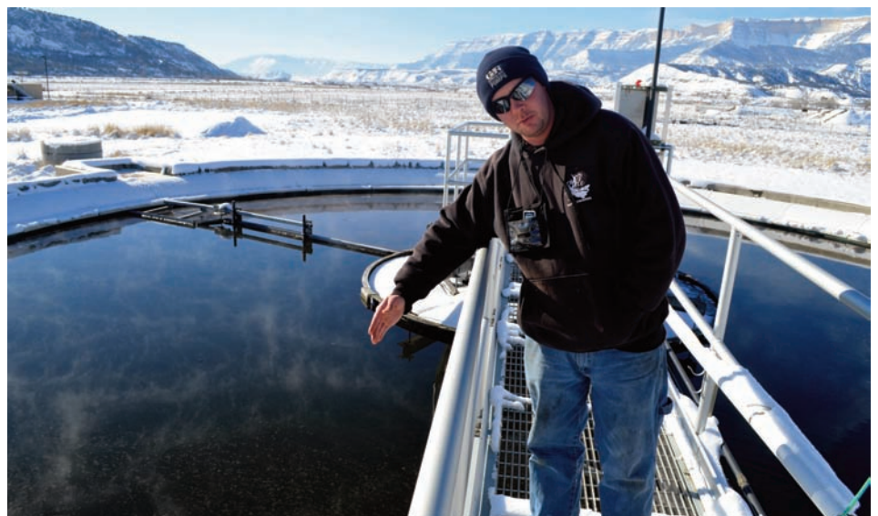
Devin Jameson of the Rifle wastewater treatment plant explains changes in the operation of the plant’s clarifiers. Photos by Cameron M. Burns
